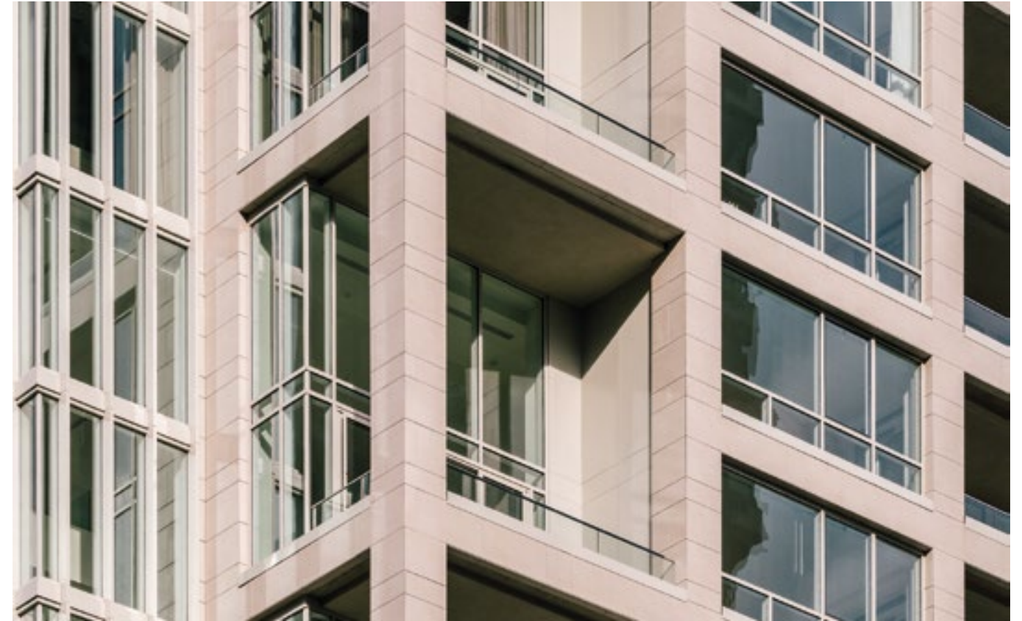
Porcelain cladding with mitered corners at The Clare Building / Manuel Glas Architect
