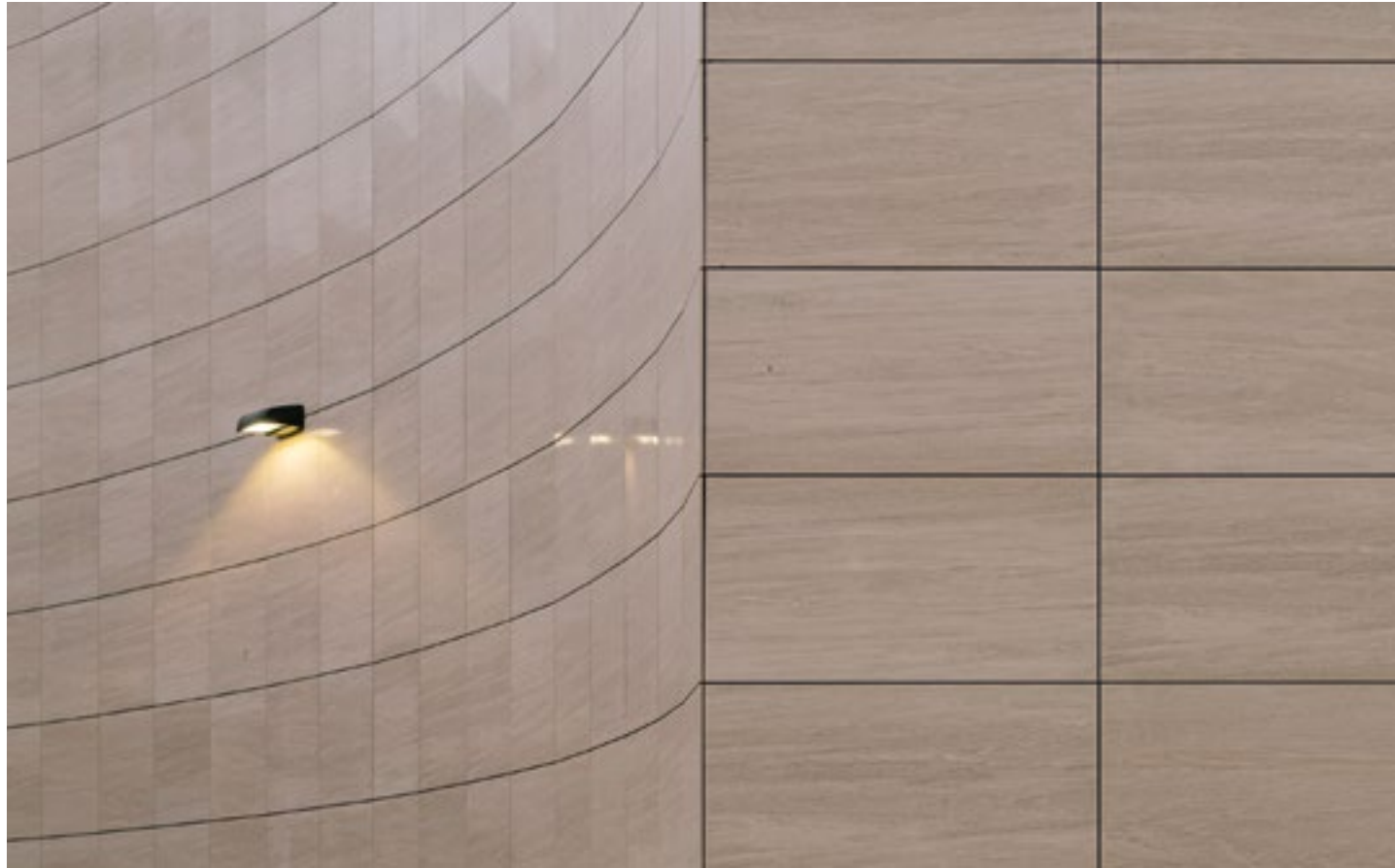
Curved porcelain cladding / AC Hotel in Cincinnati OH / CR Architecture + Design
