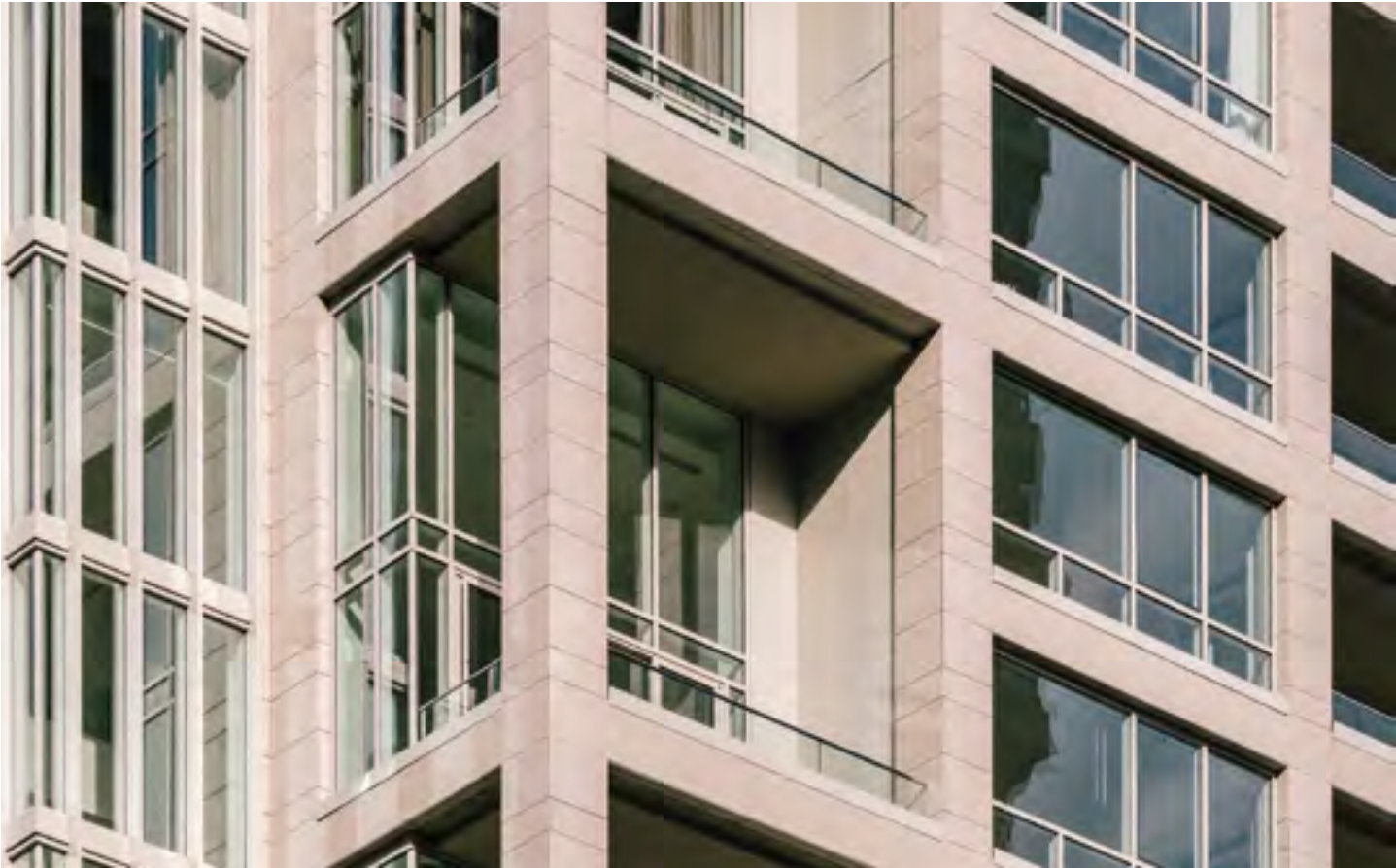
Porcelain cladding with mitered corners at The Clare Building / Manuel Glas Architect
