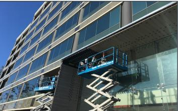
It is recommended to maintain the leveling wedges as long as possible, so that the adhesive dries. At least 24 hours. Once leveling wedges are removed, the panels can be cleaned with water and a sponge, if necessary. If there is any remaining P-404 adhesive, it can be easily cleaned with alcohol or acetone. The ventilated façade system in the soffit will also prevent the accumulation of humidity, and does not require maintenance.
