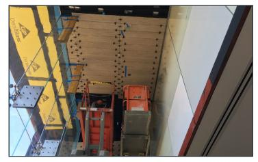
In this case, per project layout, the soffit was installed starting from center, leaving the cuts on the side.
