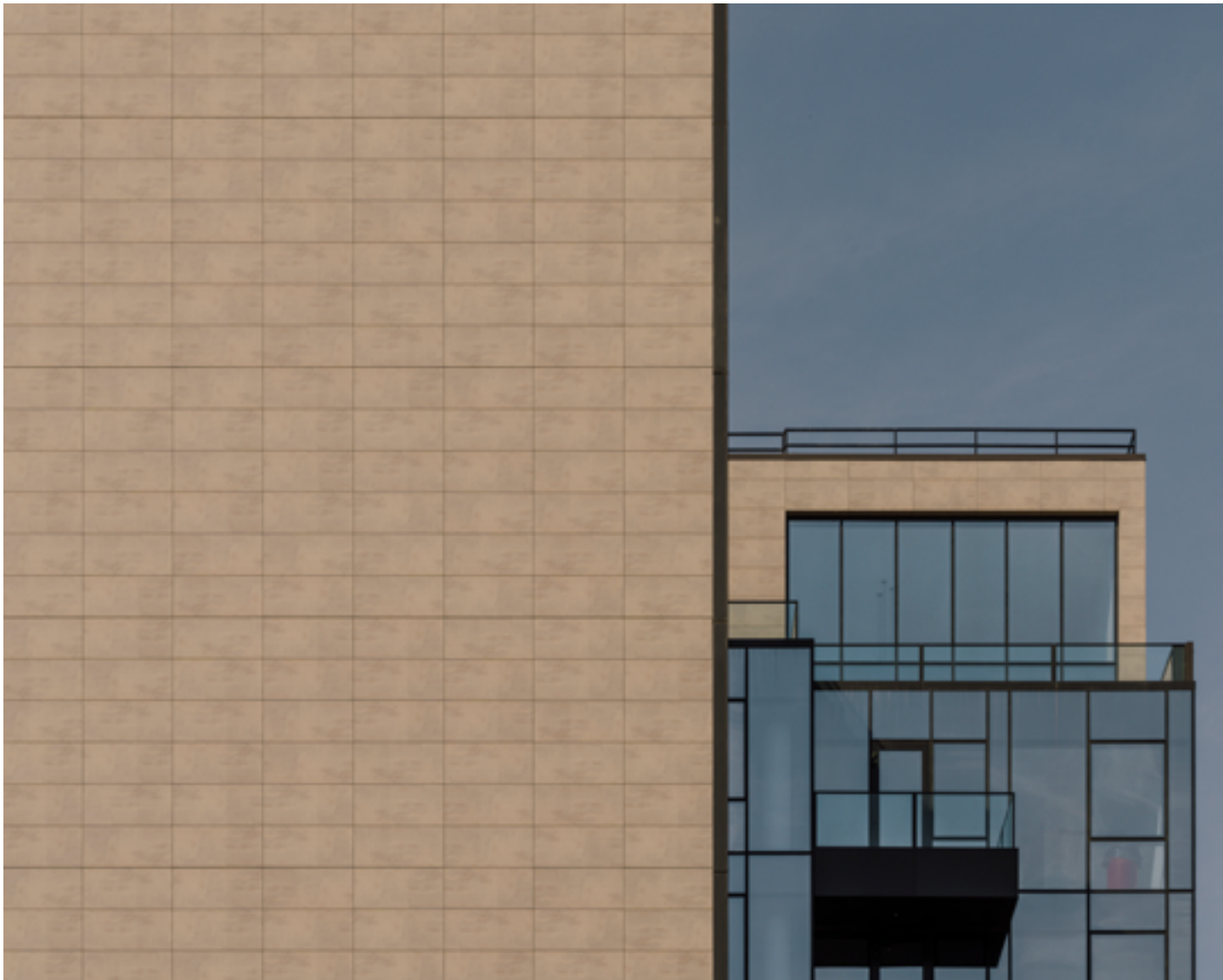
Large format porcelain wall with glass facade beyond
