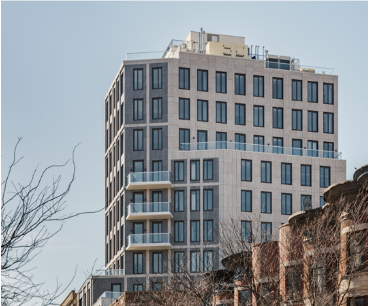
Porcelain cladding wrapping around building side facade
