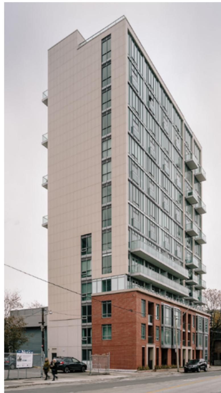
Street view of Cladded elevation and Porcelain cladding corner articulation
