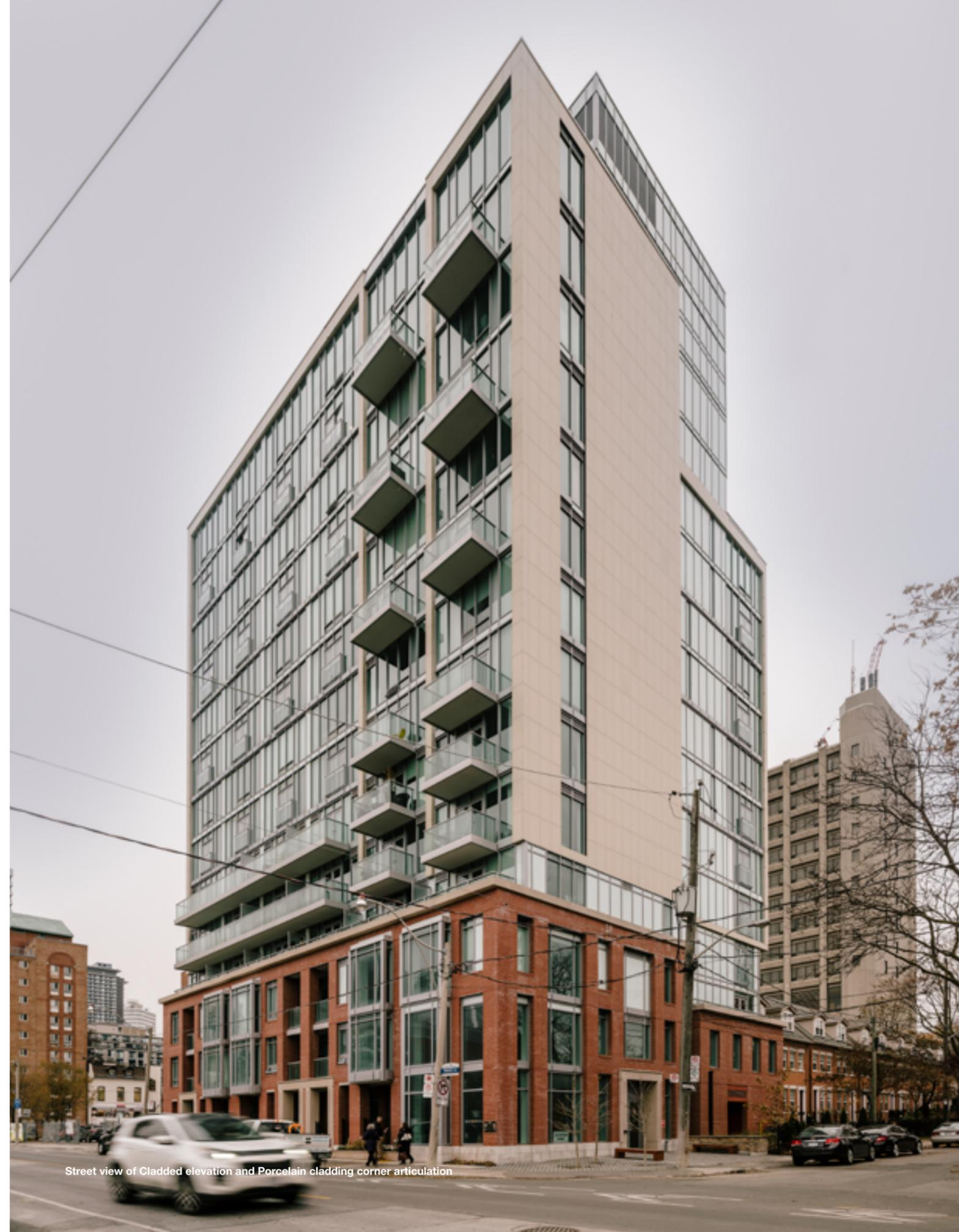
Street view of Cladded elevation and Porcelain cladding corner articulation
